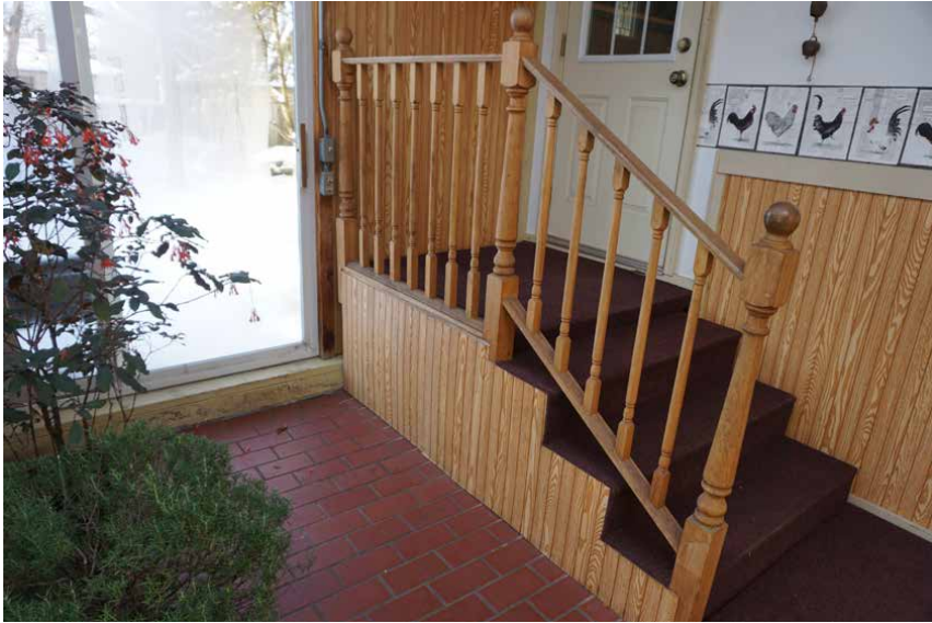
Moveable stairs cover a trapdoor to the well pit.
