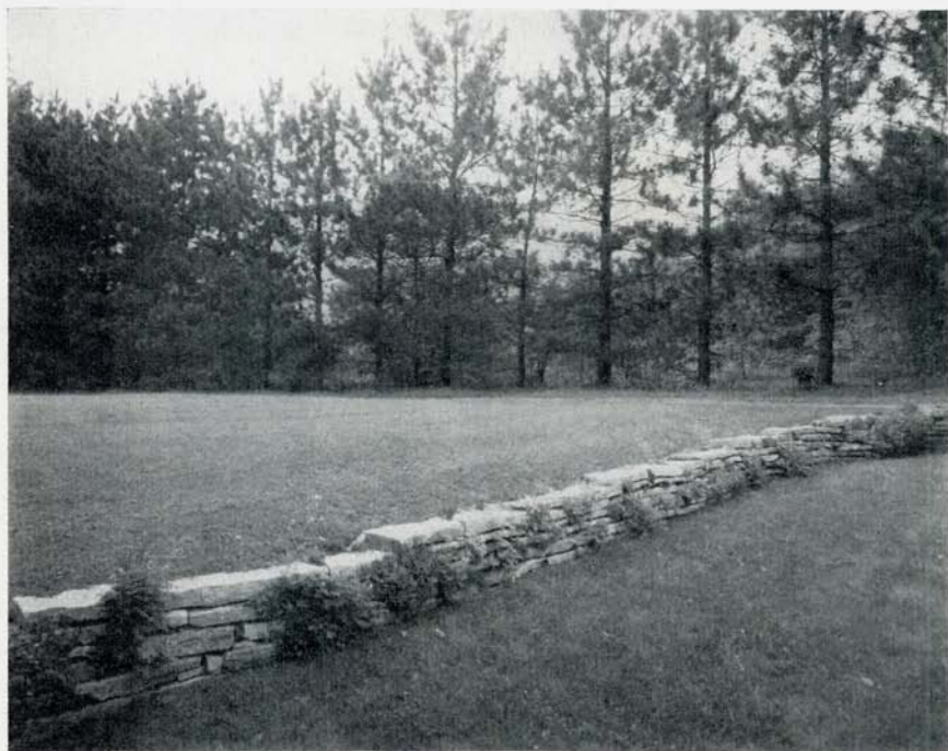
The wall: the center planted with sun lovers, while most of the face is in shade a good part of the day.
