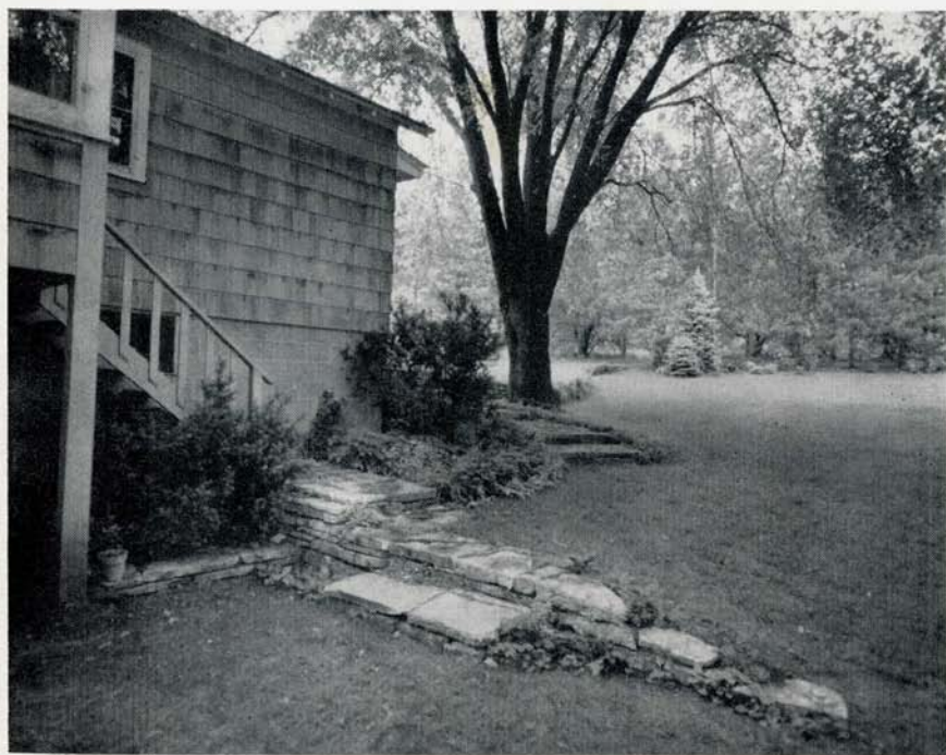
The whole project—small steps near basement entrance, stone platform by the kitchen door, planting leading to the main flight of steps, and the wall itself in the distance.
