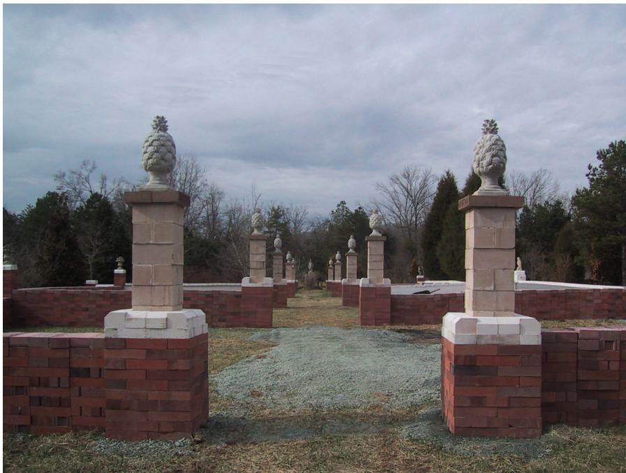
The Walled Garden under Construction
