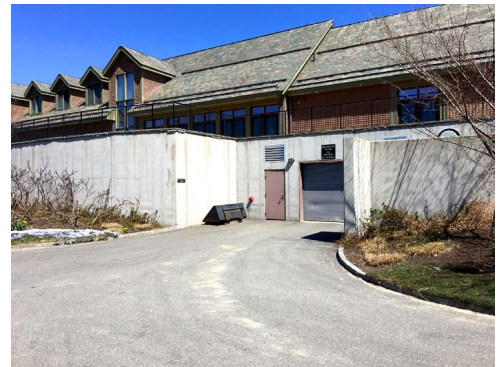
west side loading dock
