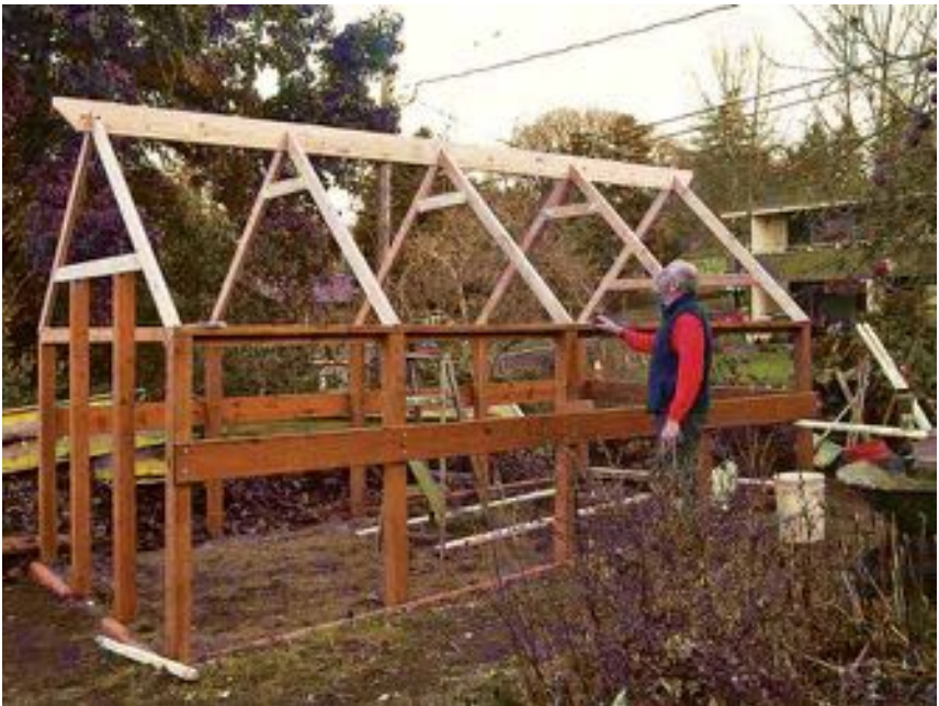
The 2 x 10-inch ridgeboard is first raised on temporary supports (above) before three pairs of rafters are put in place and the ridgeboard lowered onto them and secured. Remaining rafters are then secured in place.
