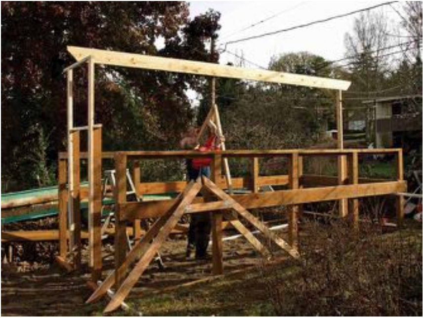
The 2 x 10-inch ridgeboard is first raised on temporary supports (above) before three pairs of rafters are put in place and the ridgeboard lowered onto them and secured. Remaining rafters are then secured in place.
